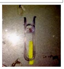
**Step 8:** Remove clip. Use a ½" drill bit and drill out the center mark. Slide the 3/8 clip back into position so the threaded part is aligned with the hole.
