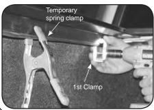
B. Hold rail in proper position with spring clamp. Install 1st clamp as close to front as possible and use 1/2" wrench to tighten.
