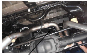
CROSS MEMBER Figure 3.2: View under bed towards axle.
