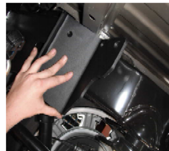
Figure 6.2: Passenger side plate looking from floor up at the passenger side frame.
