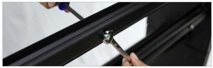
3. Tighten the nut using a 3/8" wrench and a Phillips screwdriver to hold the screw in place on the other side.
