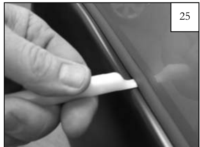
25 Using flat end of supplied Edge Trim Tool (ET1-0002), seat edge trim against flare by inserting straight end between edge trim and flare at one end. Next, slide around entire edge to the other end.
